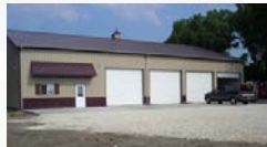
Rural fire station, northeast Kansas
